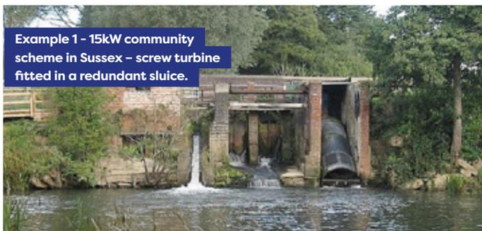
Example 1 - 15kW community scheme in Sussex - screw turbine fitted in a redundant sluice.
