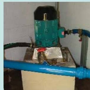
The turbine at Llanover Hydro
