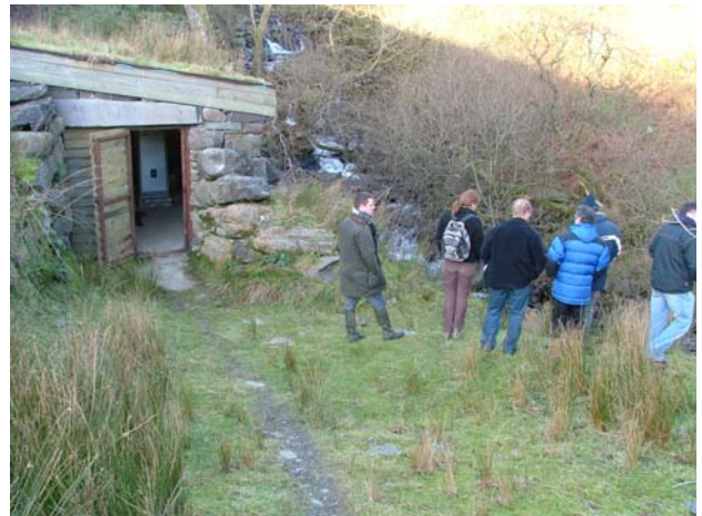
Outside the powerhouse at Maesglas
