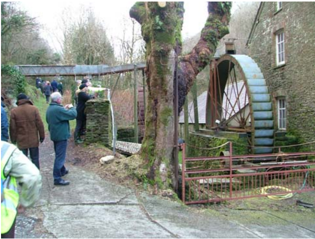
The renovated waterwheel at Dreifa Mill
