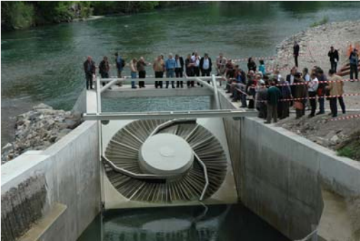
Millau Demonstration Site
