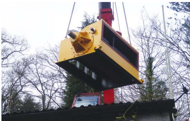
Installing the new turbine at Dolanog
