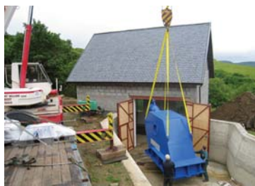
Lifting the box in
