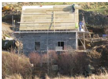
New powerhouse roof going on
